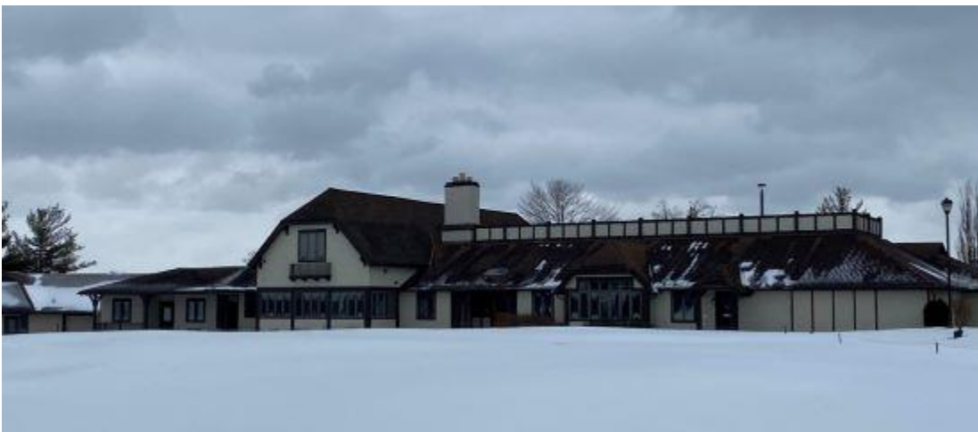
February 2022, just before demolition
